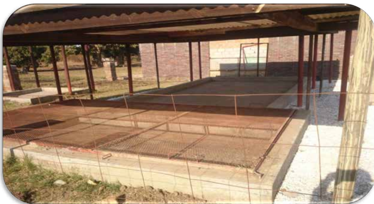
Completed DDT Evaporation tank
