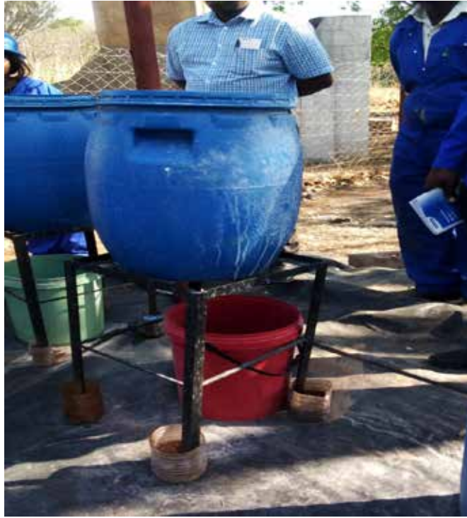
Figure 1: DDT Filtration system mounted on the stand
