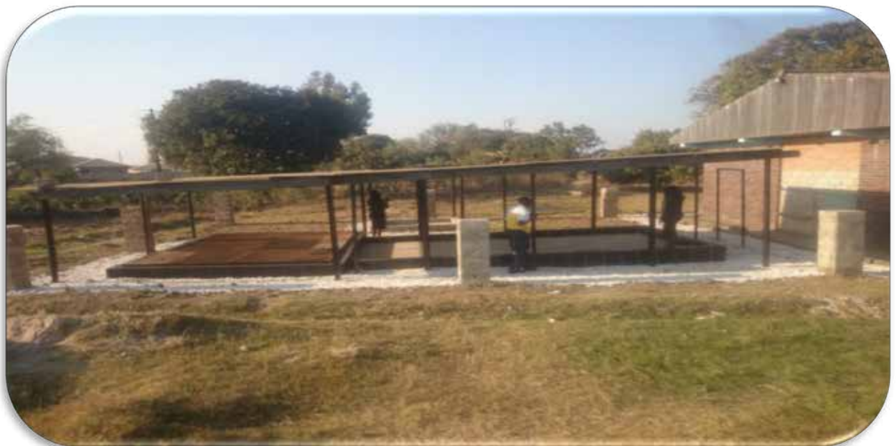
DDT evaporation tank completed and roofed
