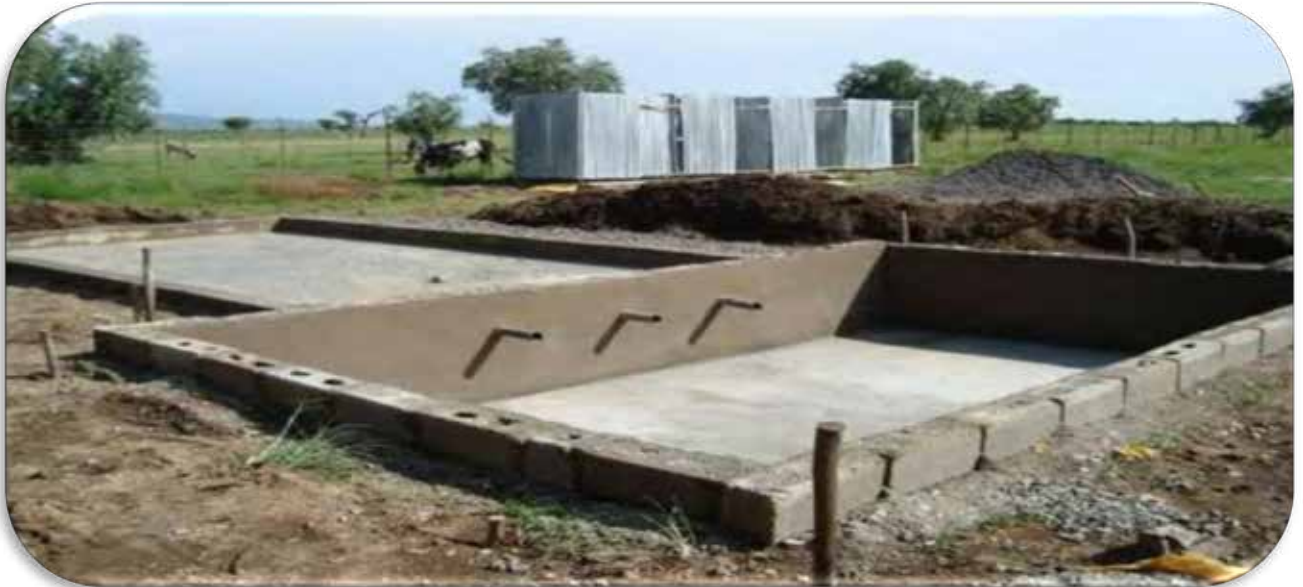
DDT evaporation tank under construction
